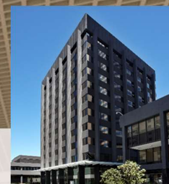
5 MILL STREET, PERTH
