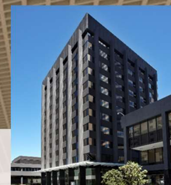
5 MILL STREET, PERTH
